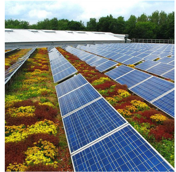
Green Roof integrated photovoltaic system
